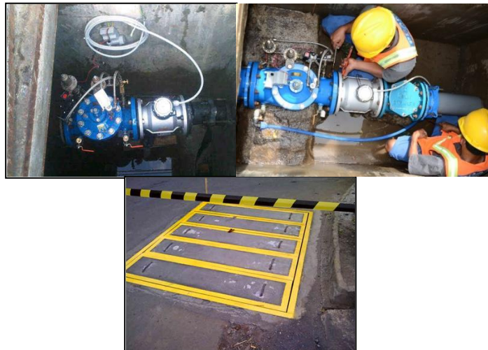
Figure 1. PRV Manhole & DMA Mother Meter
