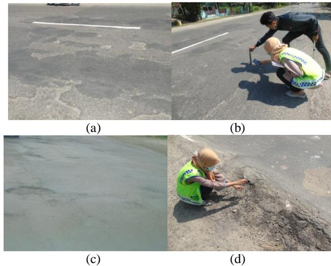
Fig. 2. Road condition identification: (a) Cracking, (b) Rutting (c), Pothole (d) Deformation.
